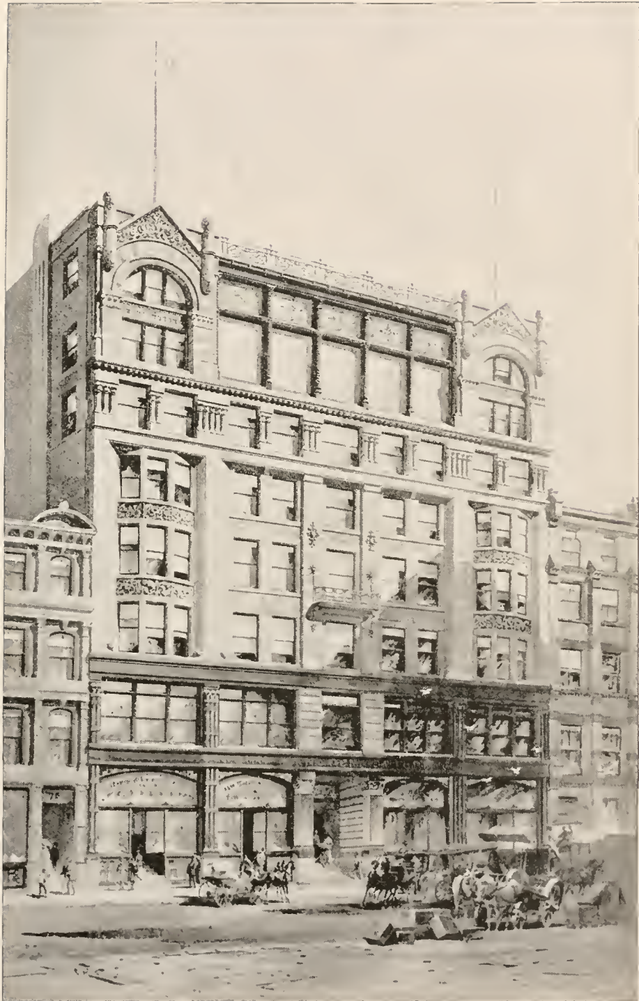
JOHN HANCOCK BUILDING.
